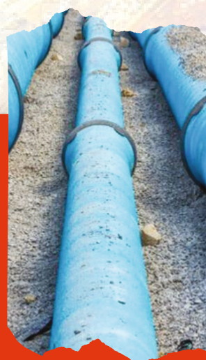
Water Pipeline Network
