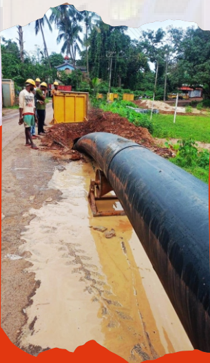
Sewer Pipeline Network
